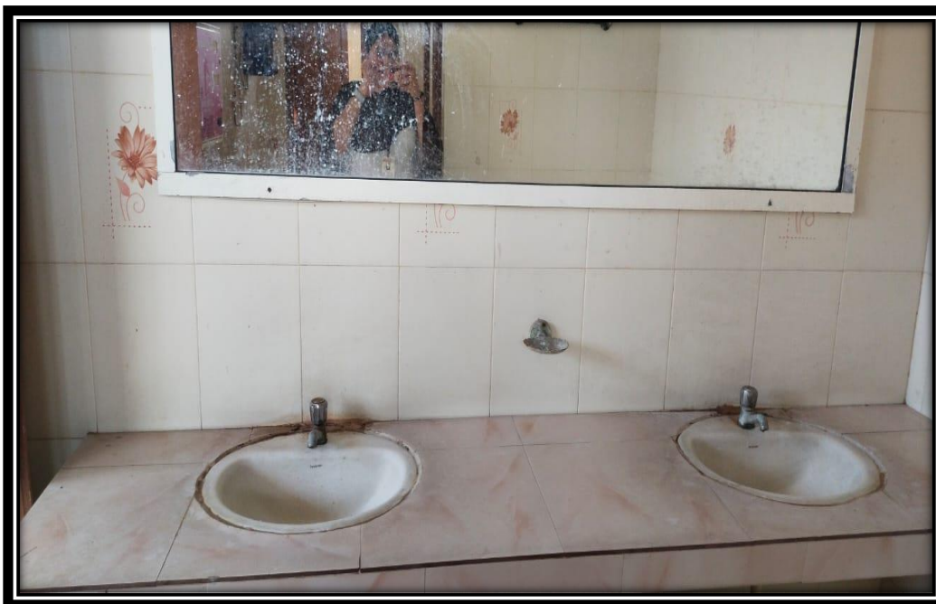
PG BLOCK - RENEWED WASH ROOMS (2017 - 18)
